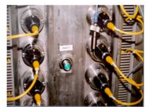
Figure 1a (Top) UV-disinfection plant for 1 800 m 3 /h in Vienna. Figure 1b (Bottom) sensor and sensor port.
